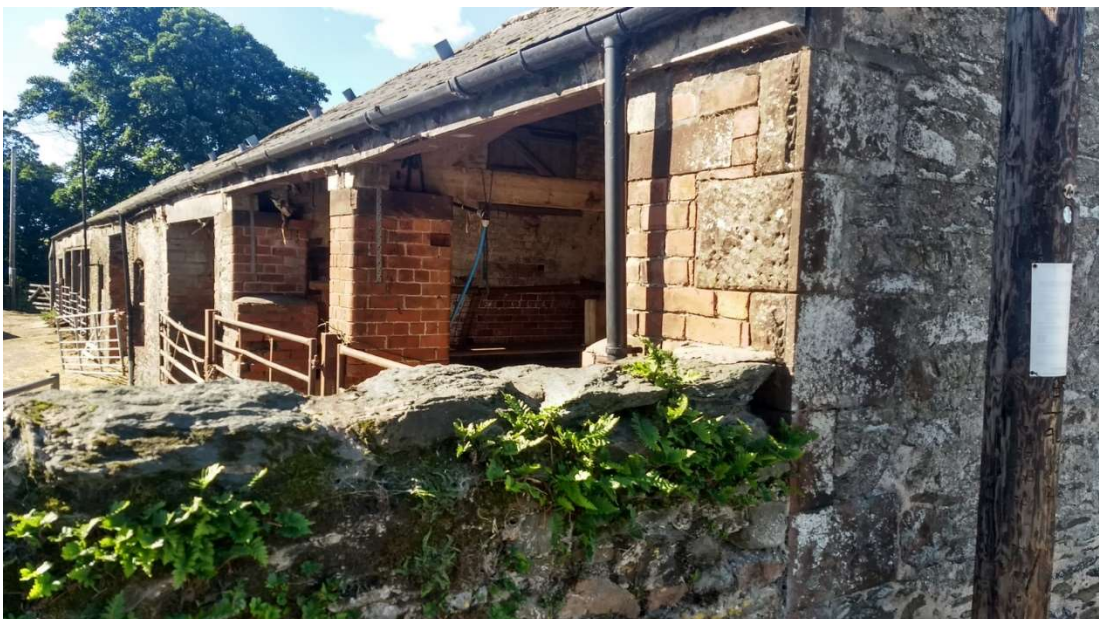
Figure 18 This old wall adjacent to the byre has small ferns growing in the top that enhance its character. Plants can, however, cause damage in masonry when left unchecked.
