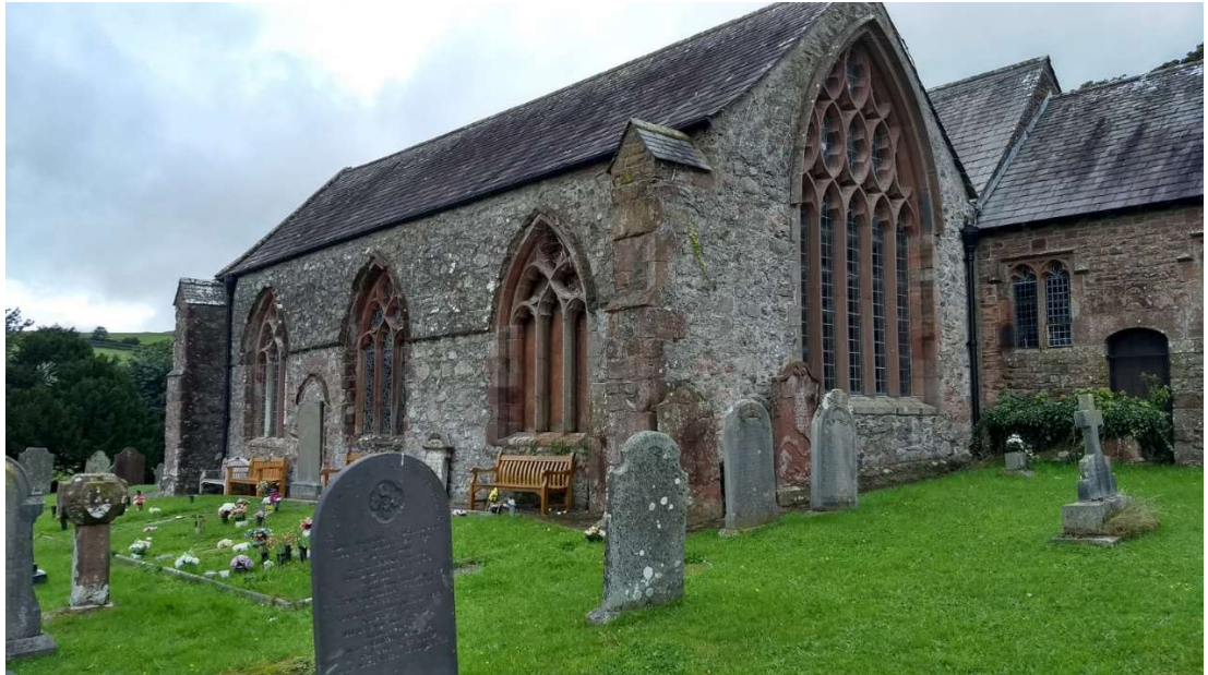
Figure 9 Holy Trinity Church from the south. The graveyard contains stones from a number of centuries, as well as a chest tomb, cross base and sundial that are listed in their own right.
